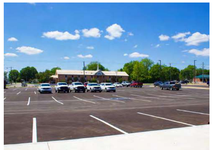
New expanded parking lot.
